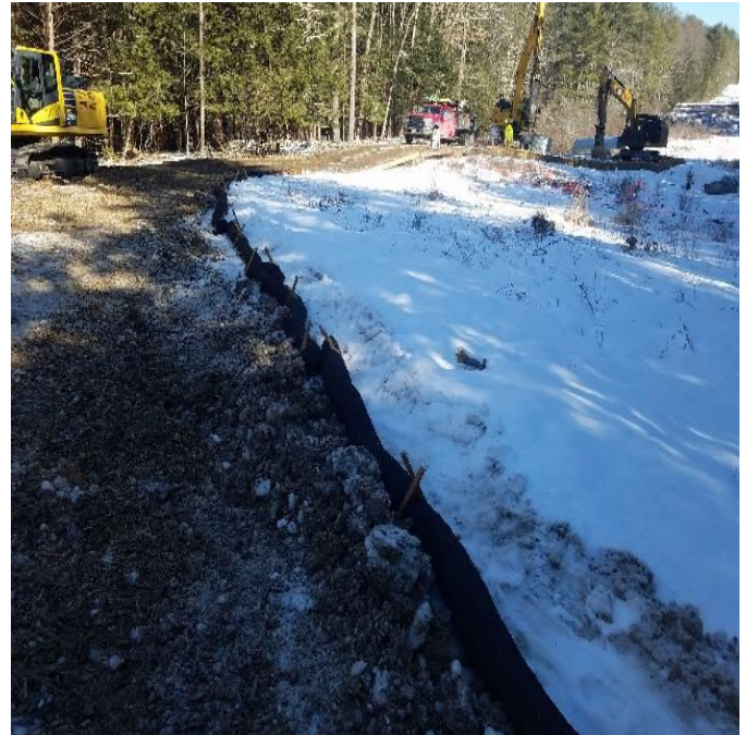
Fig 6: Filter sock installed downslope of access road to Str. 68. Viewing northeast. (02-14-20).
