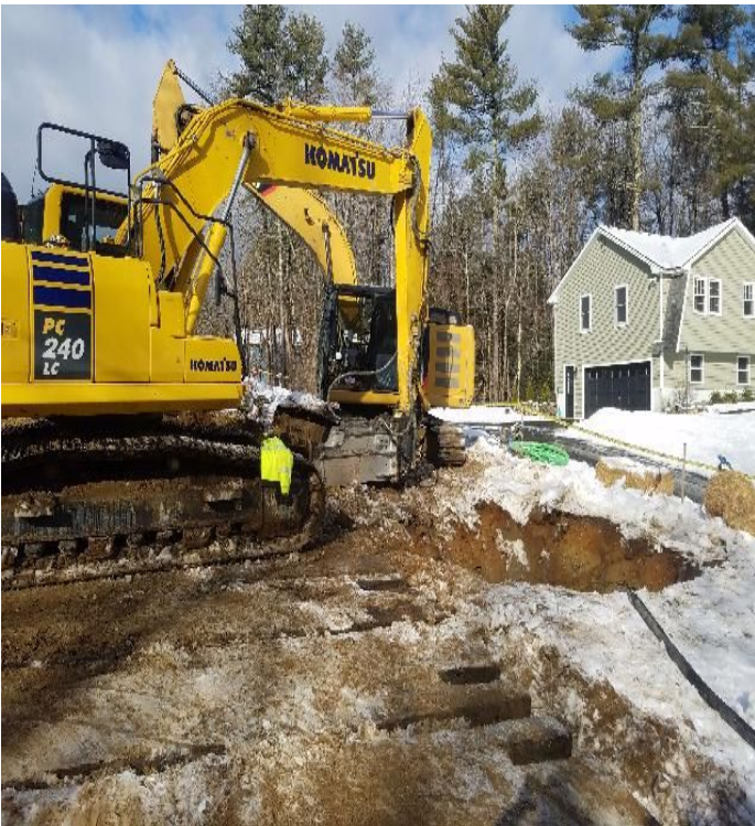
Fig 15: Excavating foundation for Str. 67. Viewing west. (02-19-20).
