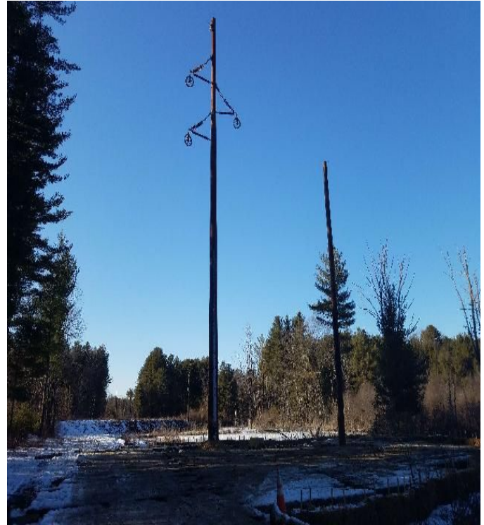
Fig 18: Str. 115 and distribution pole 3850-63. Viewing north. (02-19-20).
