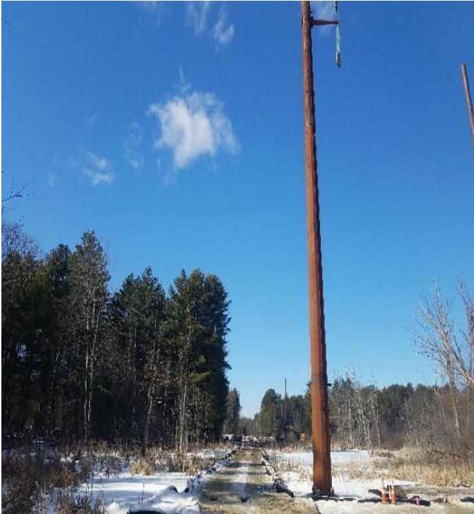
Fig 17: Str. 116. Viewing north. (02-19-20).
