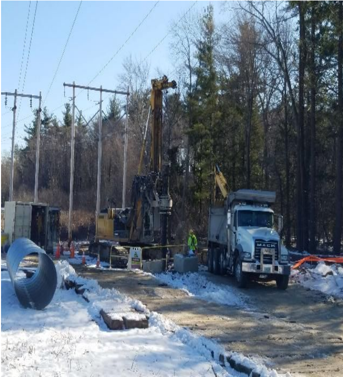
Fig 9: MJ drilling Str. 130. Viewing south. (02-14-20).
