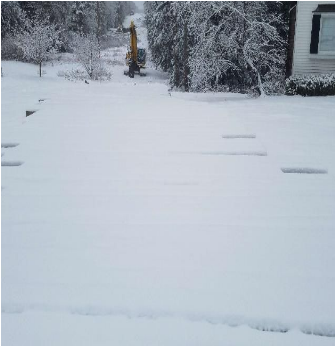
Fig 1: Access road to Str. 68, coming off of Frost Dr. Viewing east. (02-13-20).
