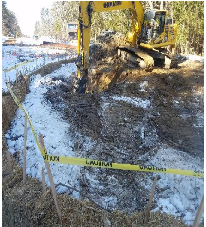
Fig 12: Crew excavating foundation for Str. 68. Viewing west. (02-17-20).
