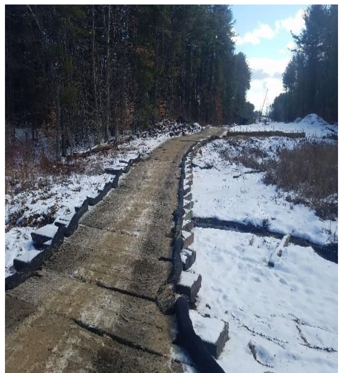
Fig 16: Access road to Str. 113 and 114, through wetland NW34. Viewing south. (02-19-20).
