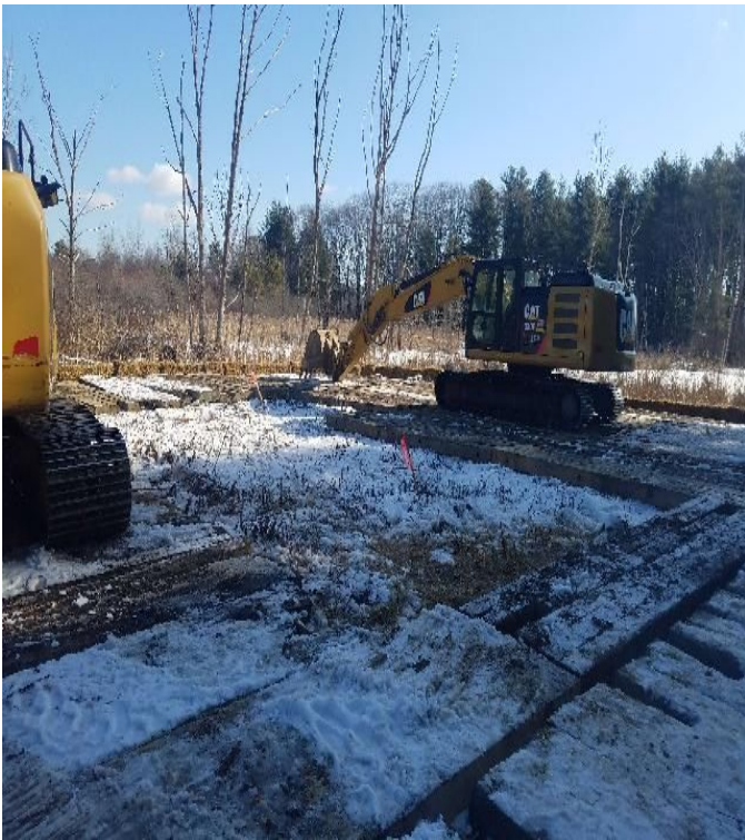
Fig 11: Str. 115 work pad. Viewing southwest. (02-17-20).
