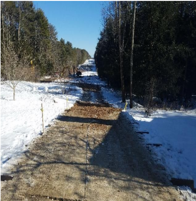
Fig 5: Access road to Str. 68. Viewing east. (02-14-20).
