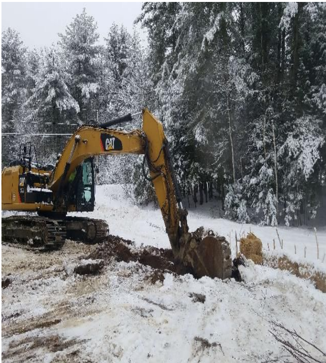
Fig 3: Crew excavating foundation for Str. 69. Viewing south. (02-13-20).
