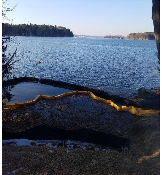
Fig 10: Turbidity barrier remains in place in intertidal zone at Gundalow landing/east side of the Bay. Viewing southwest. (02-17-20).
