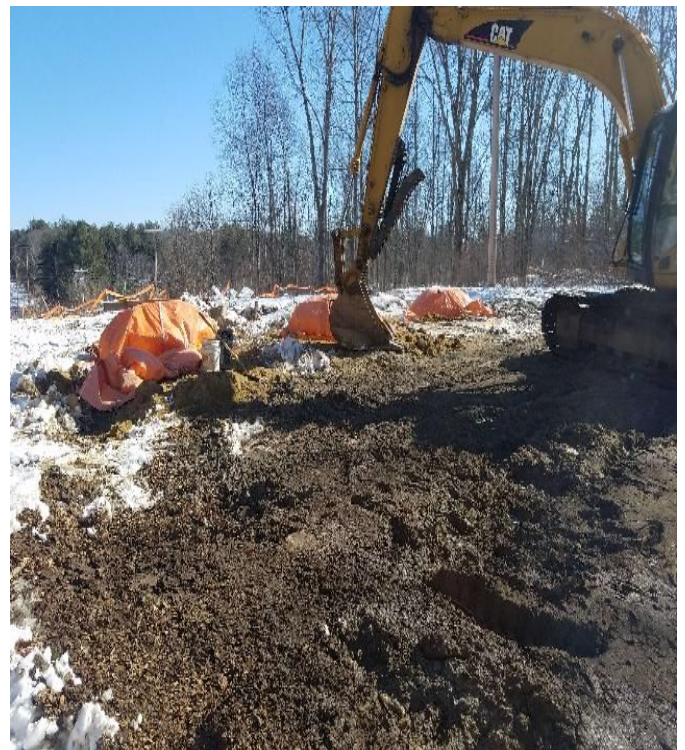
Fig 8: Crew restoring Str. 58 work area. Viewing northeast. (02-14-20).
