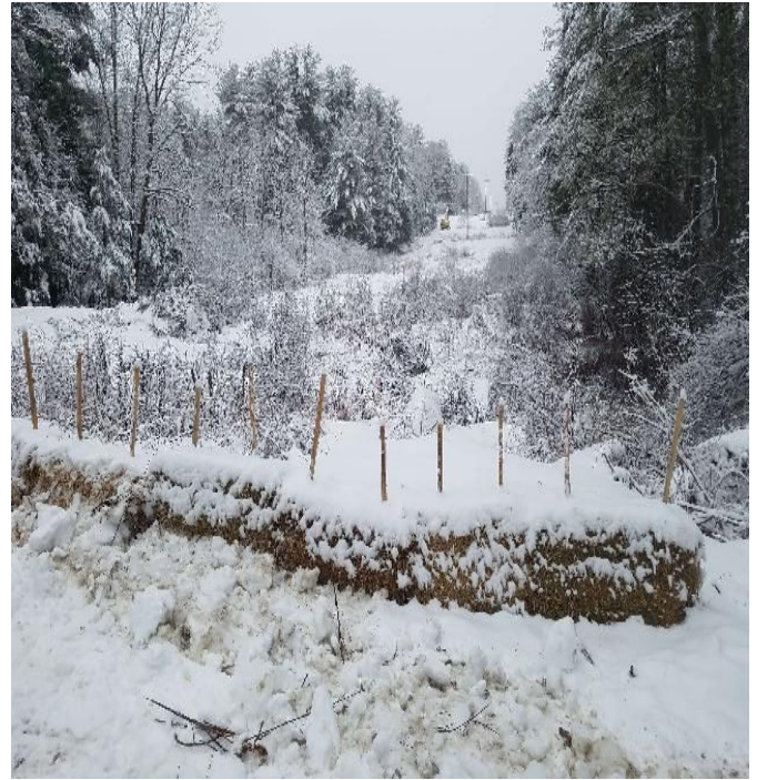
Fig 2: BMPs installed between Str. 69 work area and wetland DW13. Viewing west. (02-13-20).
